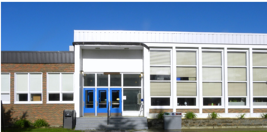
Classroom Building, Augustana Campus, Camrose, AB
