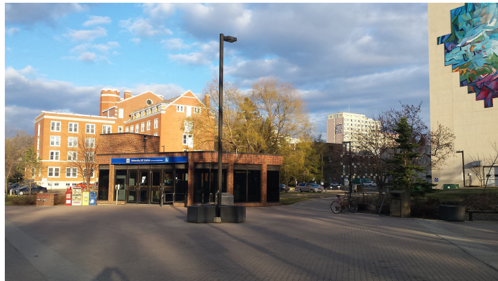
1 LRT ENTRANCE TO UNIVERSITY STATION
