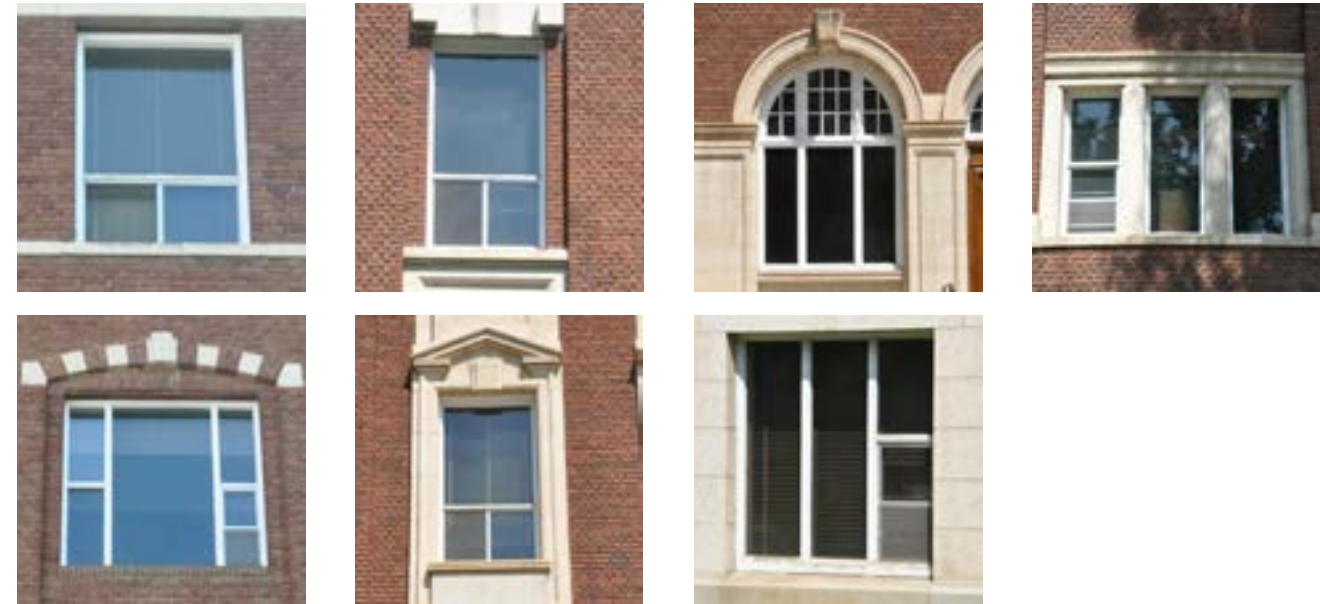
Figure 86 - Window Types - 1922 Building
