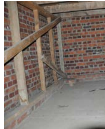
F. Attic with slab floor
