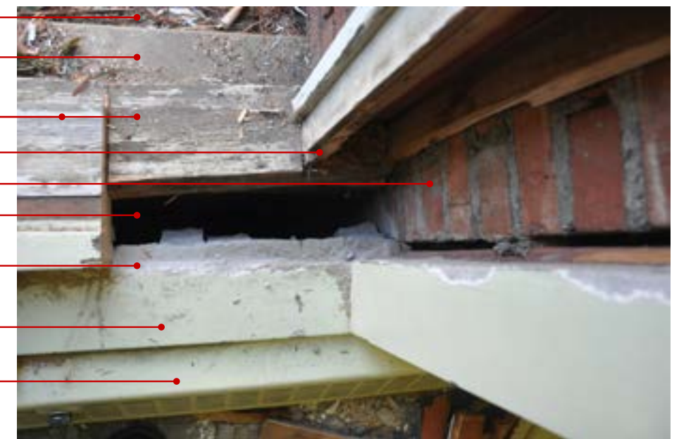
Figure 16 - 1922 Window - Jamb looking at Sill
