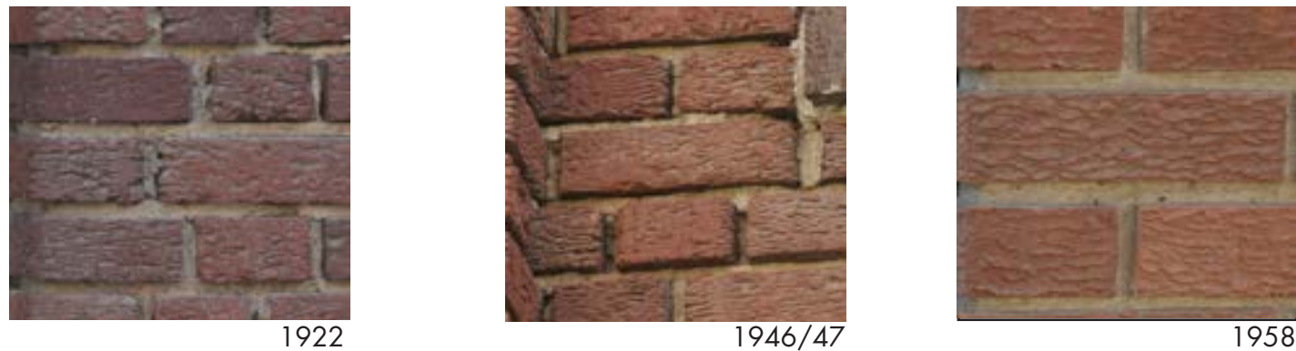
Figure 5 - Existing Brick Masonry Types/Condition
