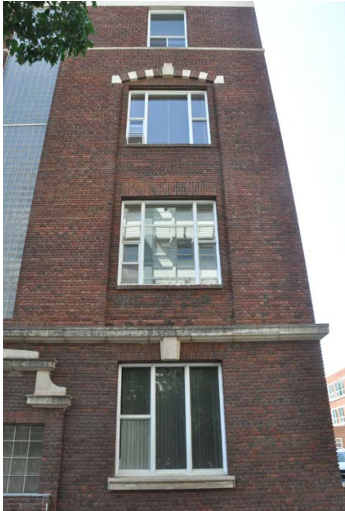
Figure 24 - 1946 Windows - North Elevation West Wing
