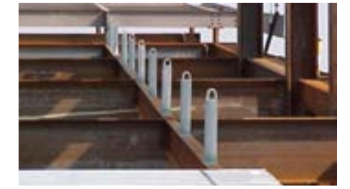
Roof Anchor Welded
