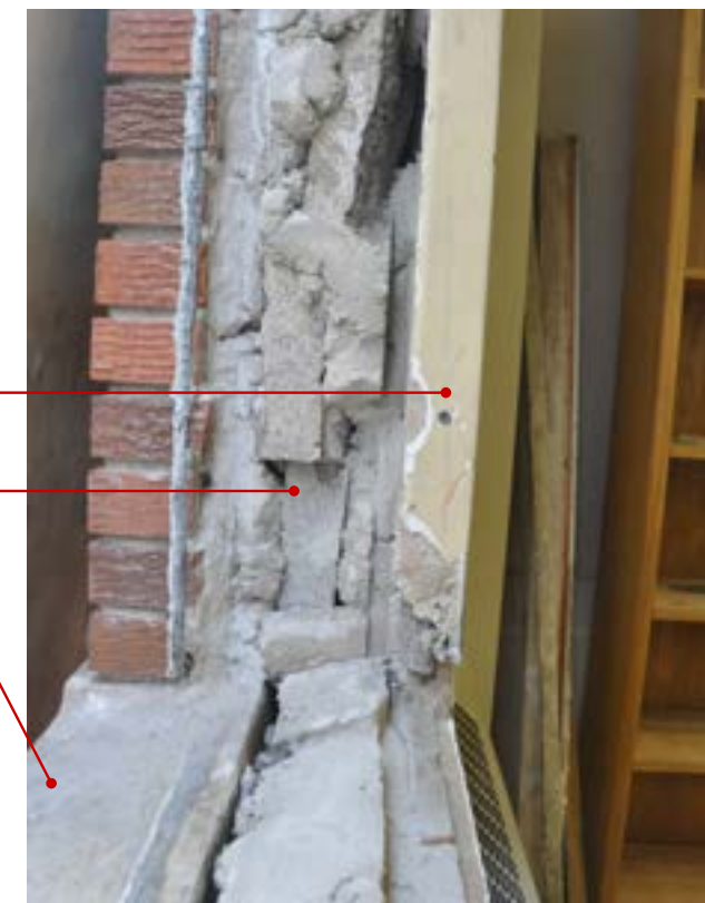
Figure 46 - 1958 Window - Sill and Jamb
