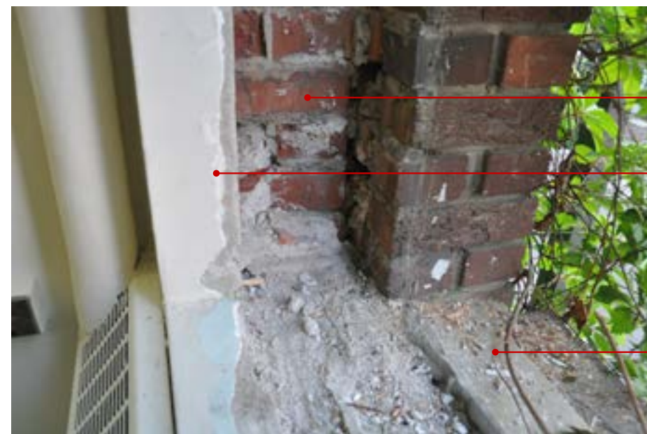
Figure 35 - 1946 Window - Sill at Jamb - exposed
