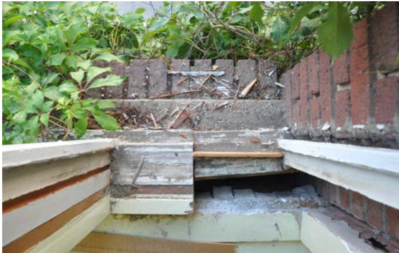
Figure 2 - 1922 Selective Demolition - West Facade
