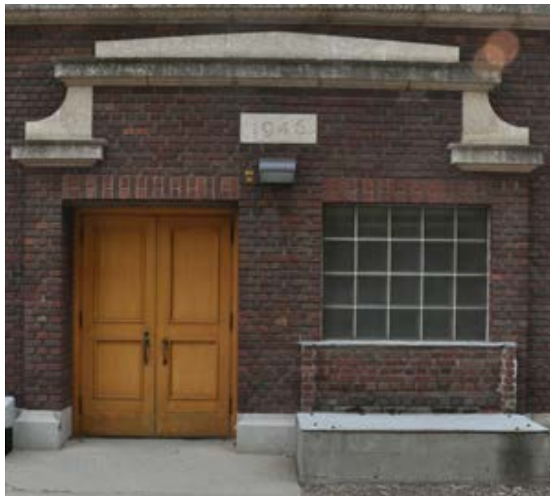
Figure 10 - 1946 - North-West Stair Entrance
