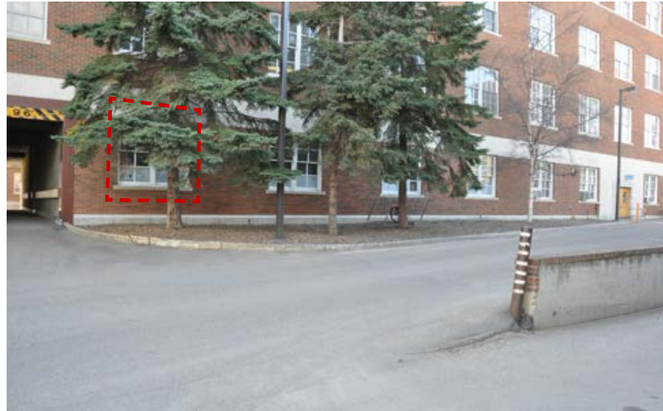
Figure 4 - 1958 Window Investigation Location (North Elevation)
