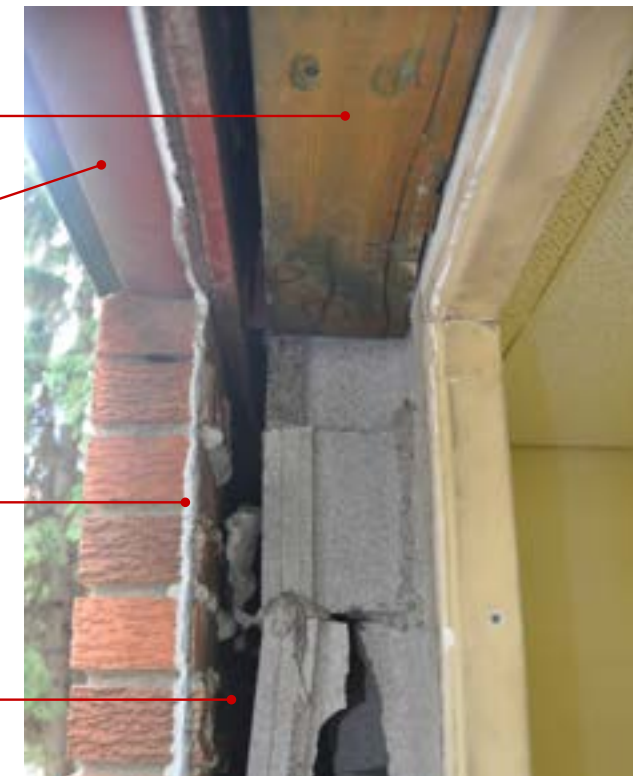
Figure 45 - 1958 Window - Head and Jamb
