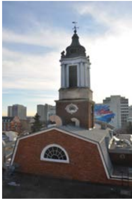
Figure 77: 1922 Cupola and Gambrel Roof
