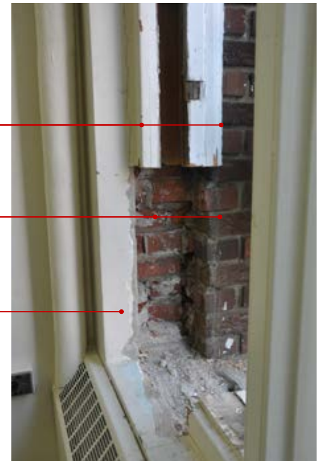
Figure 31 - 1946 Window Jamb exposed at Sill
