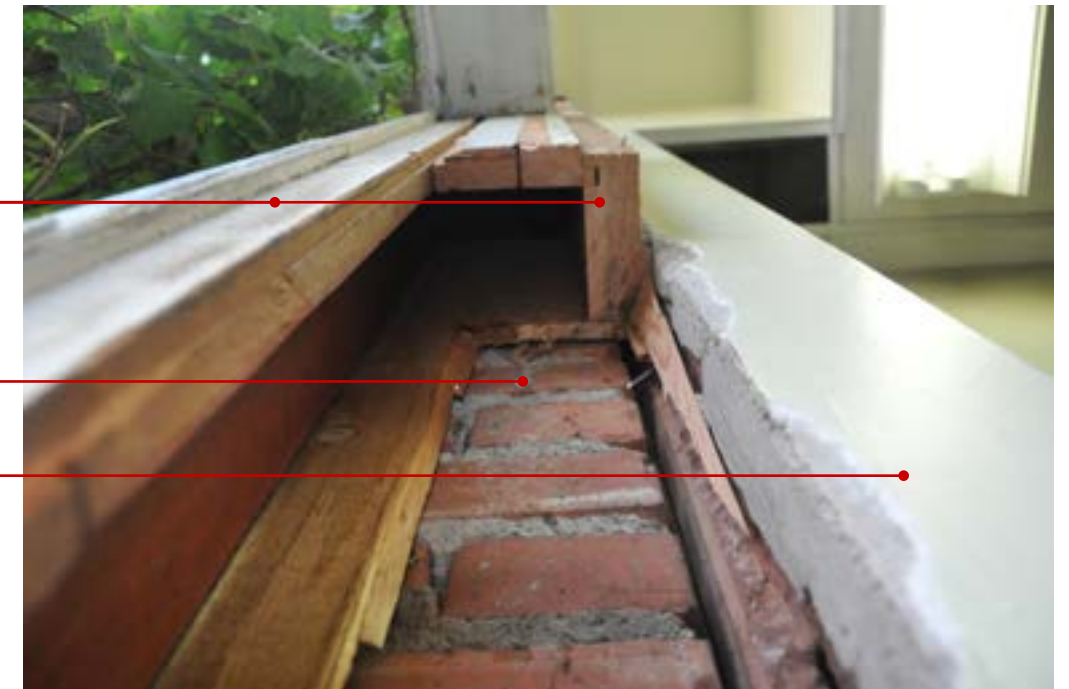
Figure 21 - 1922 Window - Jamb looking at Head
