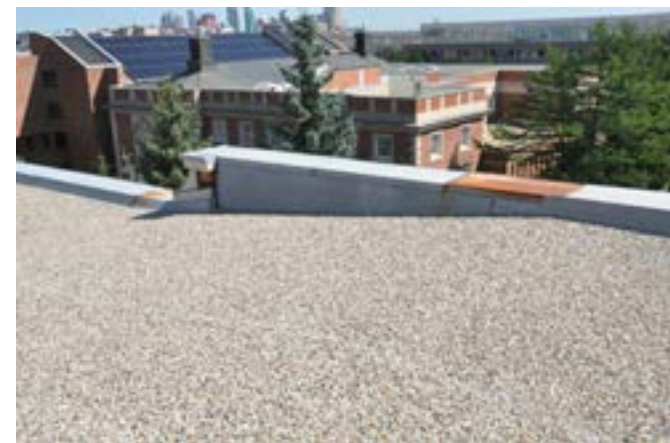
Figure 63: 1922 Parapet - East Side
