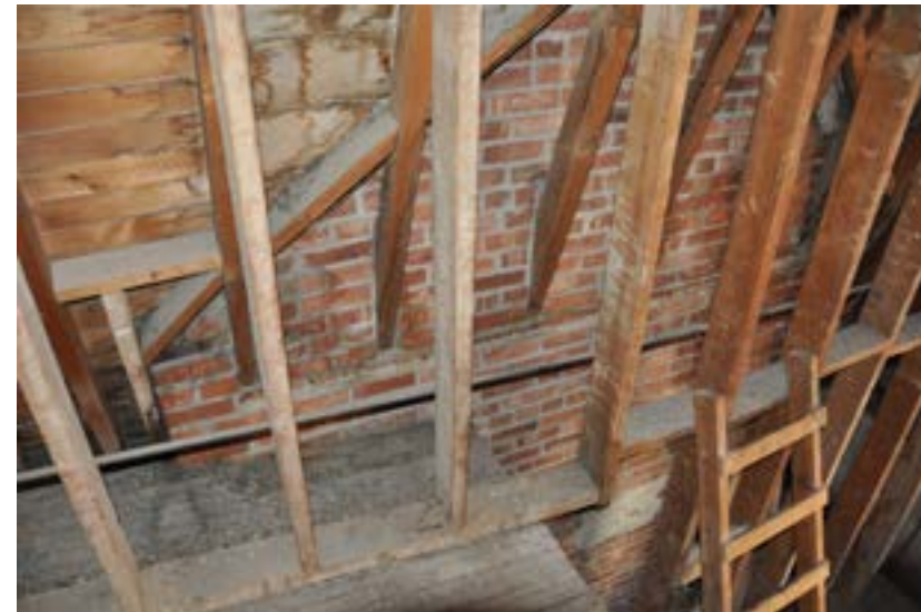
H. Mechanical Penthouse Gambrel Roof
