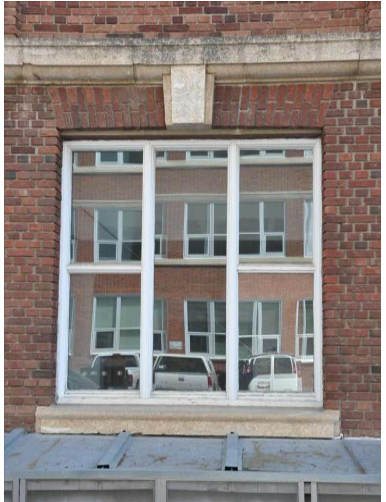
Figure 25 - 1946 Windows - West Elevation West Wing
