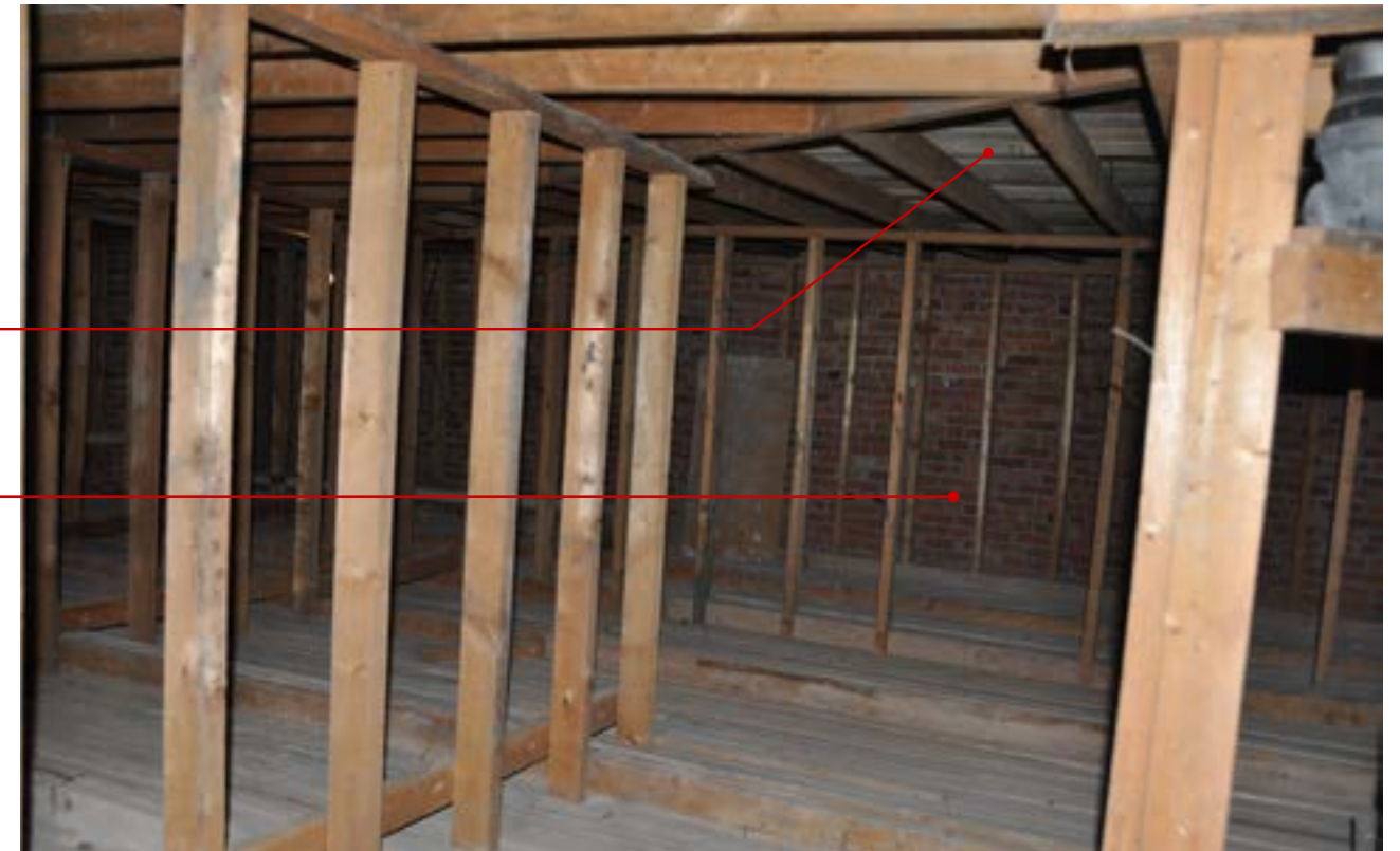
Figure 54: 1922 Typical Attic Space
