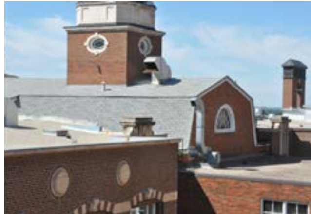
Figure 78: 1922 Gambrel Roof
