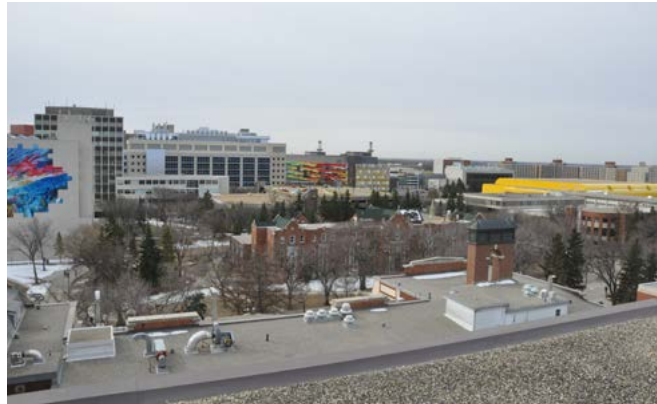
Figure 58: 1922 South West Roof
