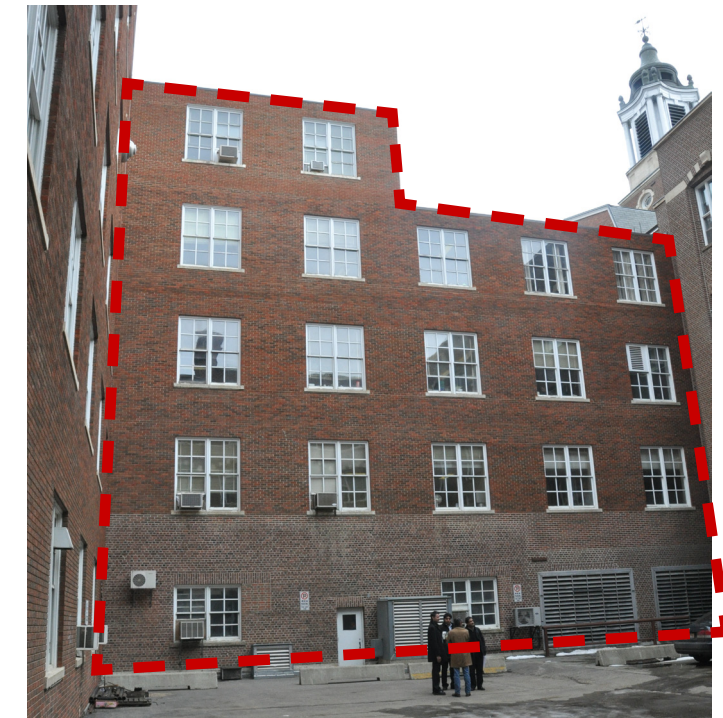
Centre Wing from West Courtyard
