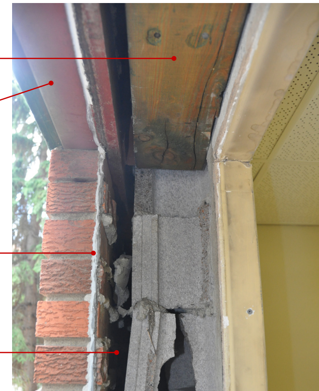
Figure 45 - 1958 Window - Head and Jamb
