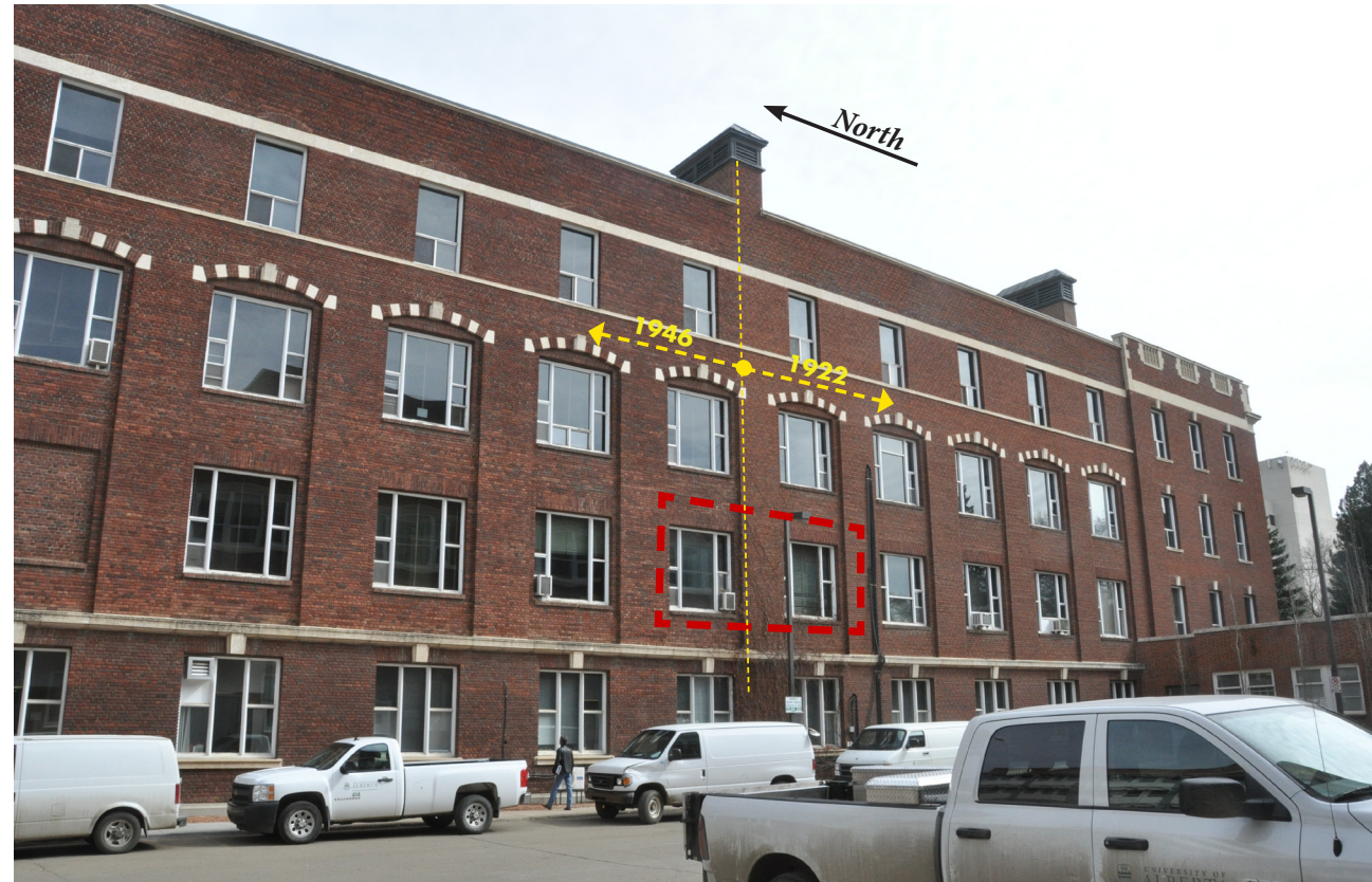
Figure 3 - 1922/1946 Window Investigation Locations (West Elevation)
