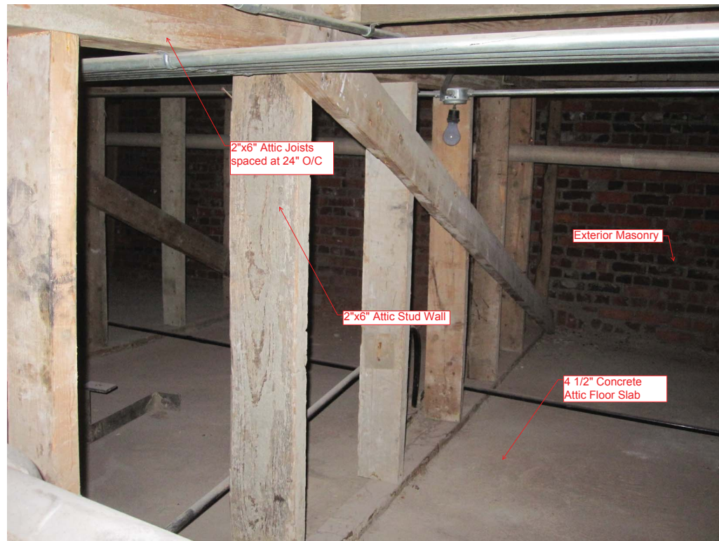
Picture of 1946/1947 Attic Space
