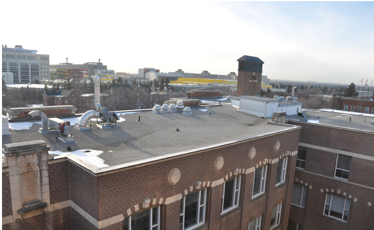
Figure 56: 1922 South West Rooftop
