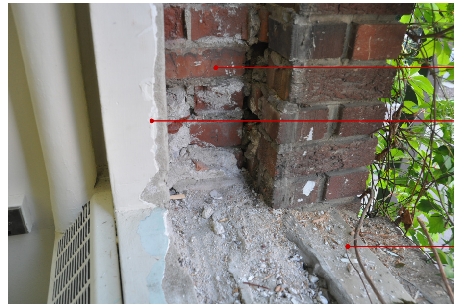
Figure 35 - 1946 Window - Sill at Jamb - exposed
