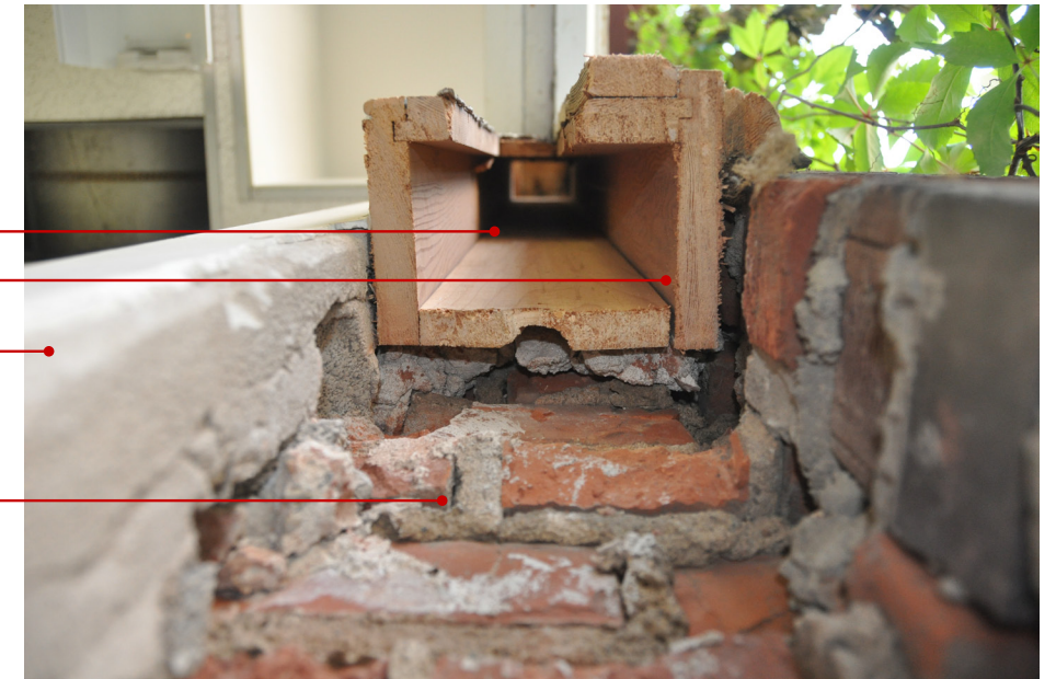
Figure 30 - 1946 Window - Jamb - Pully box frame looking up at Head
