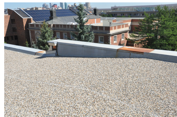
Figure 63: 1922 Parapet - East Side
