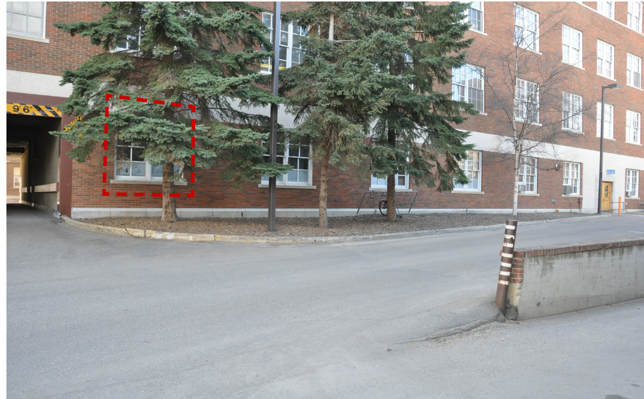
Figure 4 - 1958 Window Investigation Location (North Elevation)
