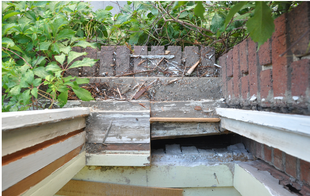
Figure 2 - 1922 Selective Demolition - West Facade
