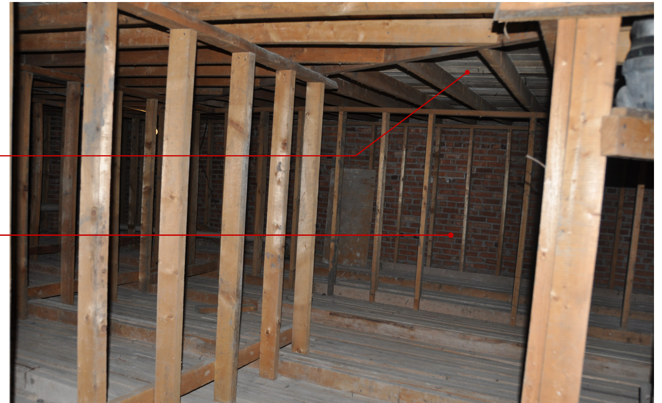
Figure 54: 1922 Typical Attic Space
