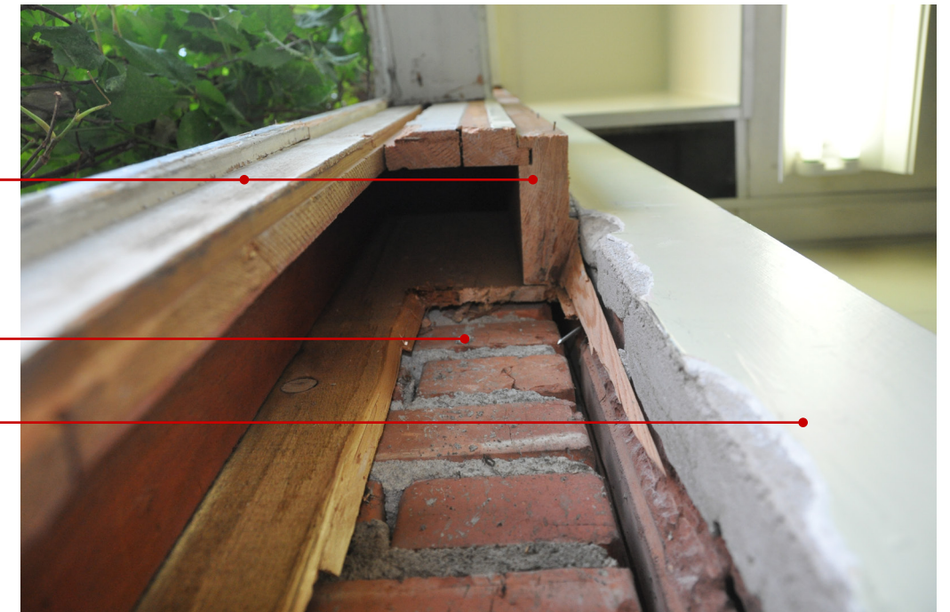
Figure 21 - 1922 Window - Jamb looking at Head
