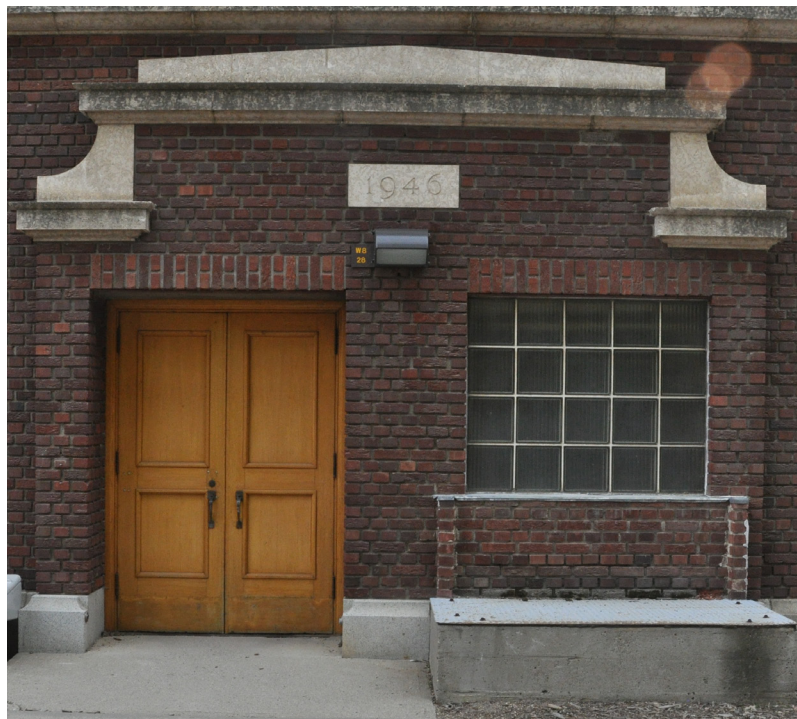
Figure 10 - 1946 - North-West Stair Entrance
