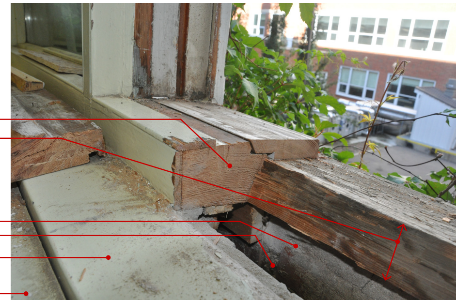
Figure 19 - 1922 Window - Level 2 Sill
