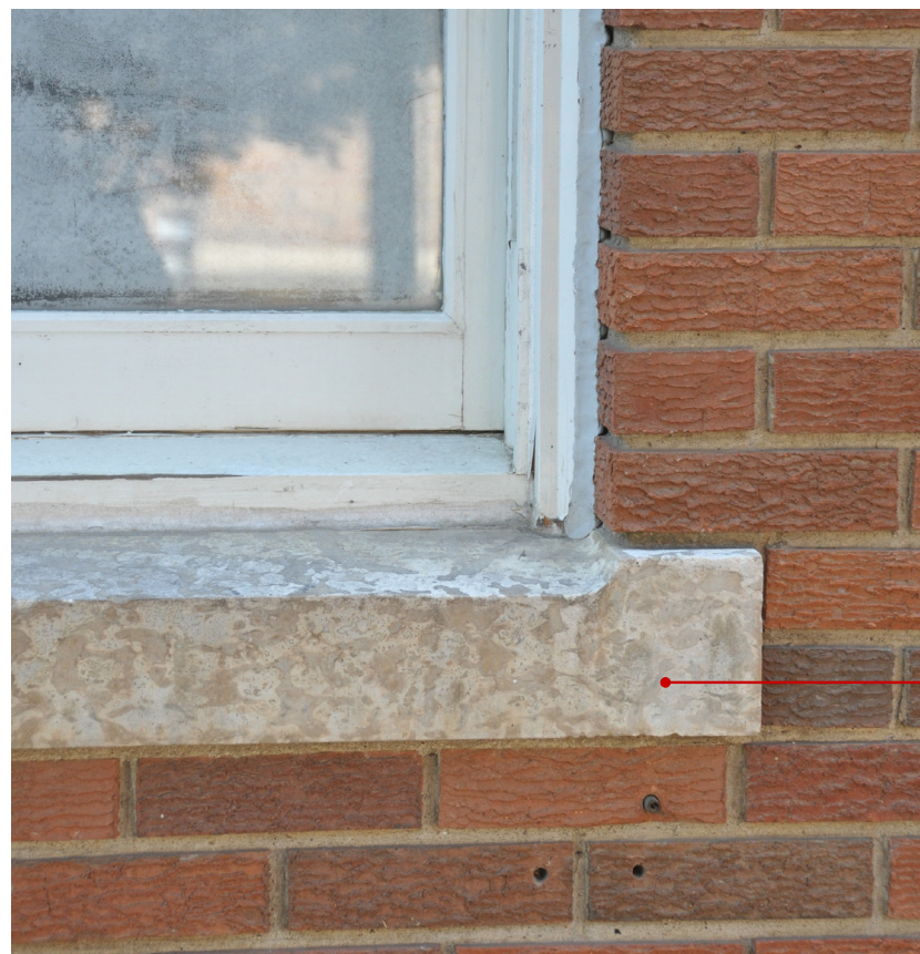
Figure 47 - 1958 Window - Sill Elevation
