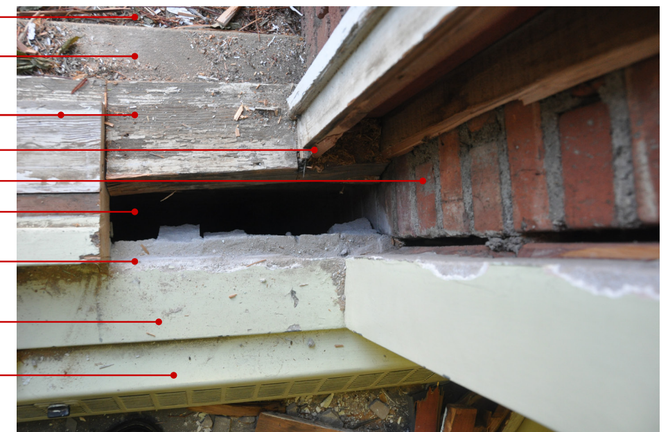
Figure 16 - 1922 Window - Jamb looking at Sill
