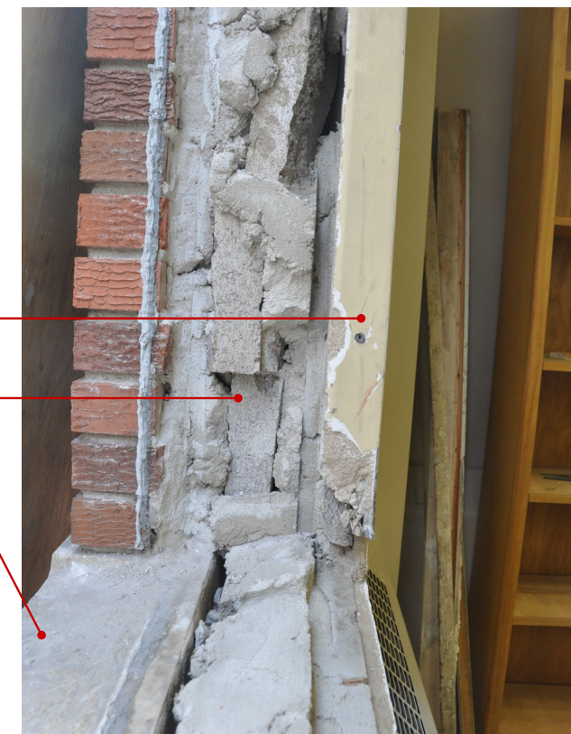
Figure 46 - 1958 Window - Sill and Jamb
