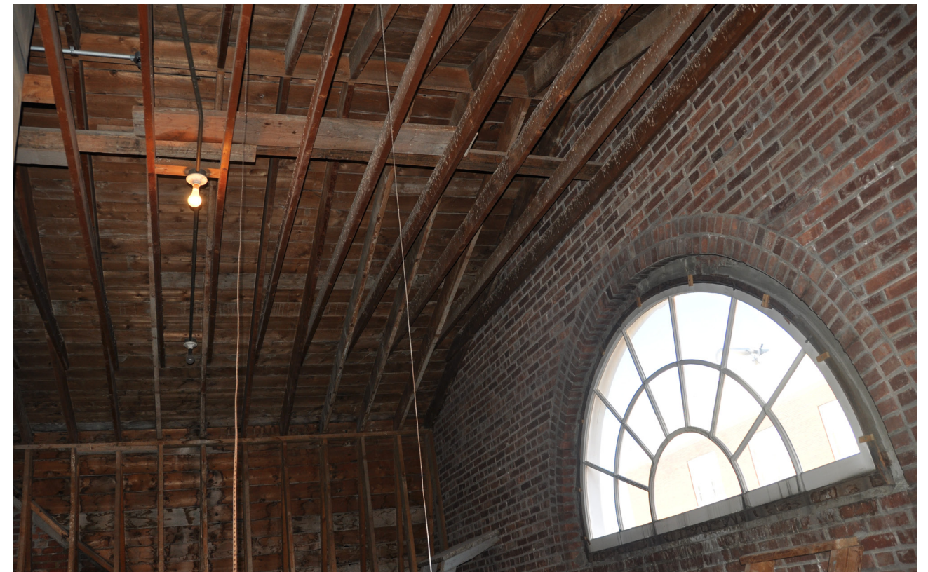
Figure 55: 1922 Mechanical Room - Gambrel Roof
