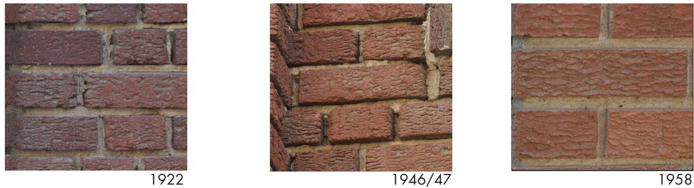
Figure 5 - Existing Brick Masonry Types/Condition
