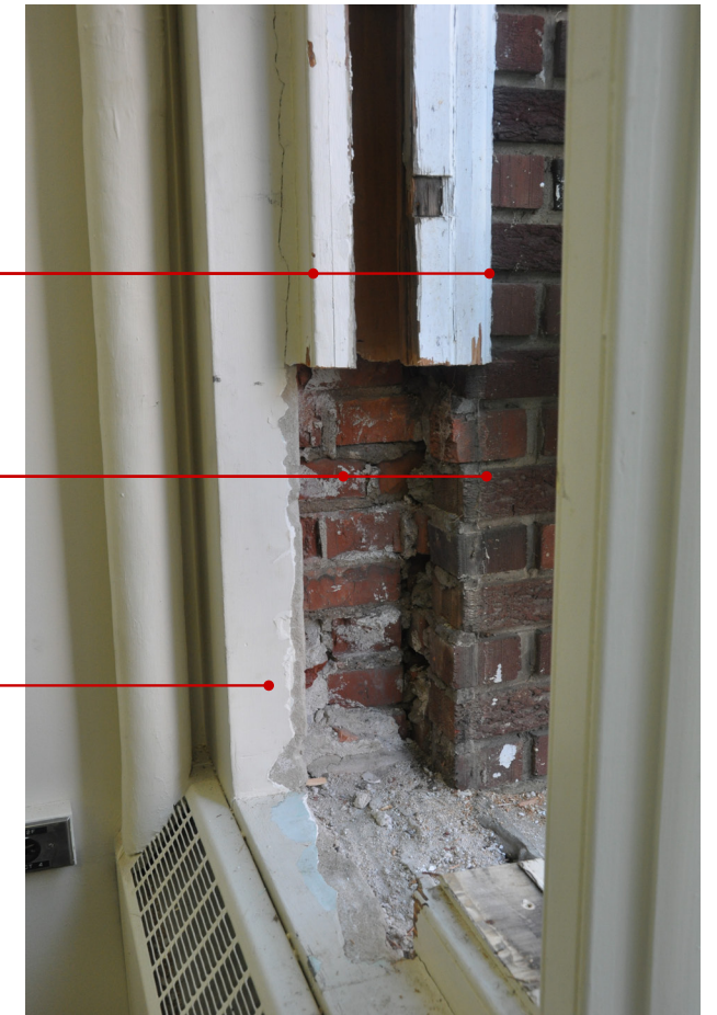
Figure 31 - 1946 Window Jamb exposed at Sill
