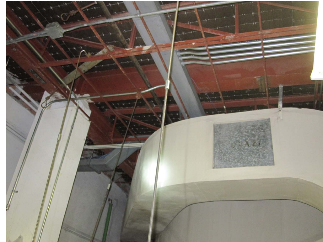
Picture of 1958 Roof Construction
