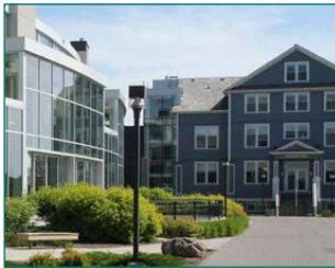
Renovation of Founders' Hall
