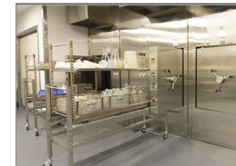
Autoclave Repair Core
