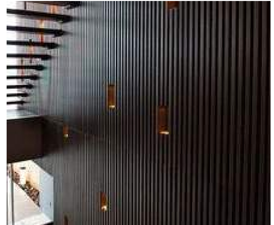
Black slatted walls will cover the side and rear walls of the chamber. The slats provide the opportunity for different backings to suit the acoustic needs of the space.
