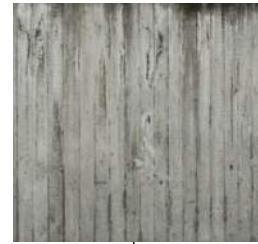
boardform concrete columns
